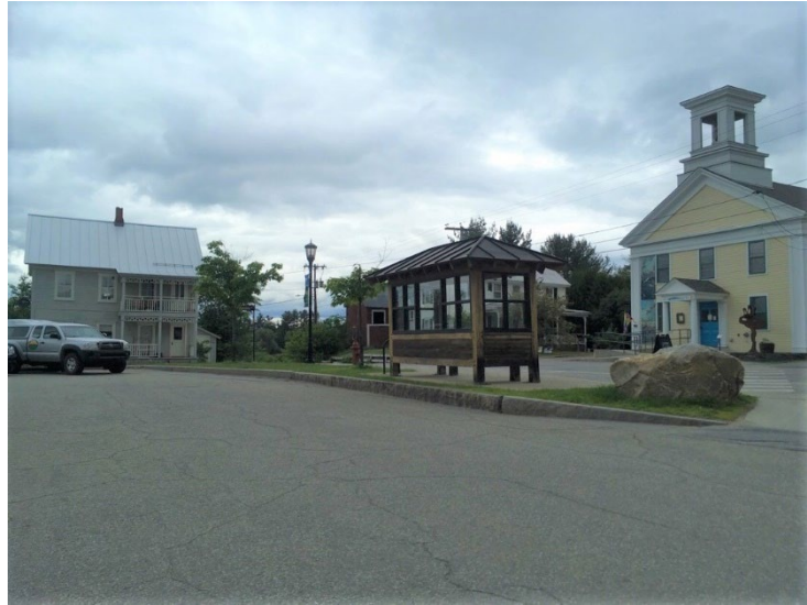
Figure 9. Subsurface infiltration chambers are proposed in the parking lot by the corner of Pleasant St and Hutchins St.
